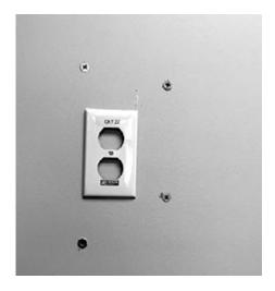
HINT: If you use an electric drill with a Phillips driver head, make sure the head fits the anchor perfectly, as the anchor or screw can strip easily. Set the drill to a slow rotation.
